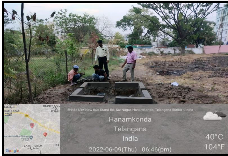
Construction of rain water harvesting pits
